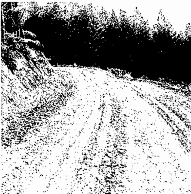
Figure 17 - A typical spur road
