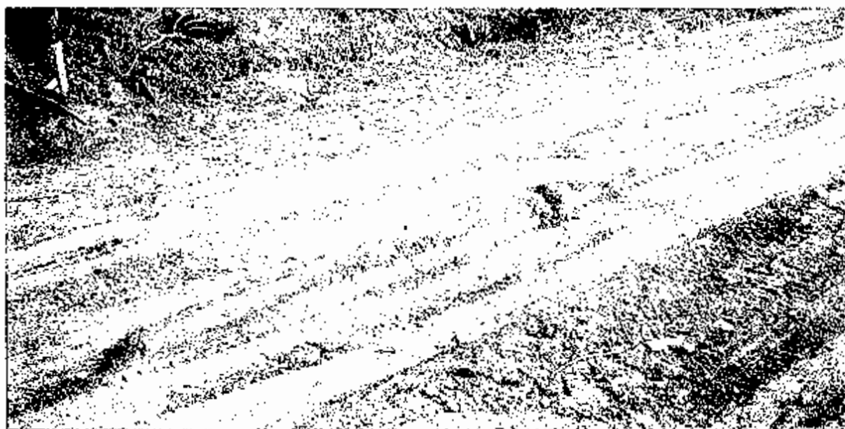
Figure 134 - Rutted pavement
