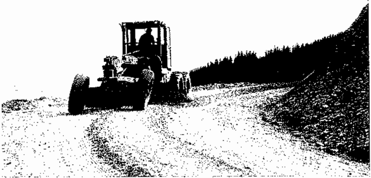
Figure 135 - Grader re-shaping road pavement
