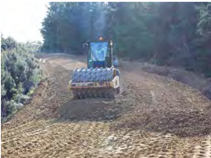
Compaction needs to be done in layers
