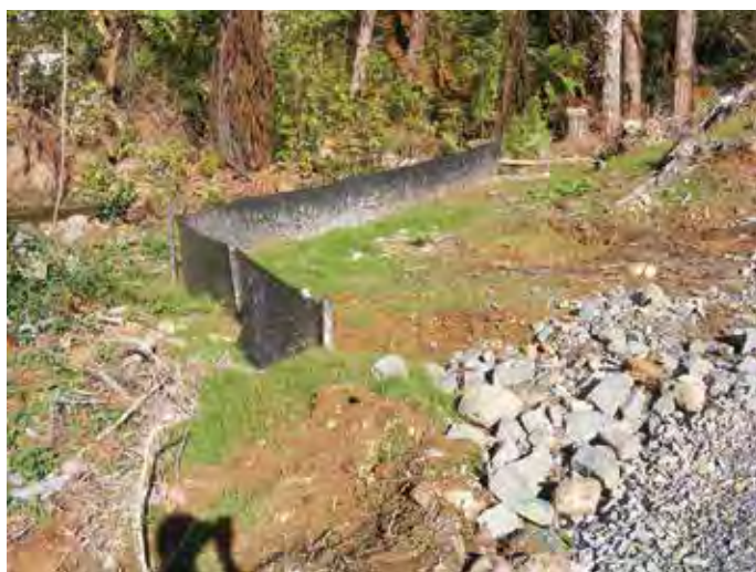
Two well-constructed applications for sediment fences
