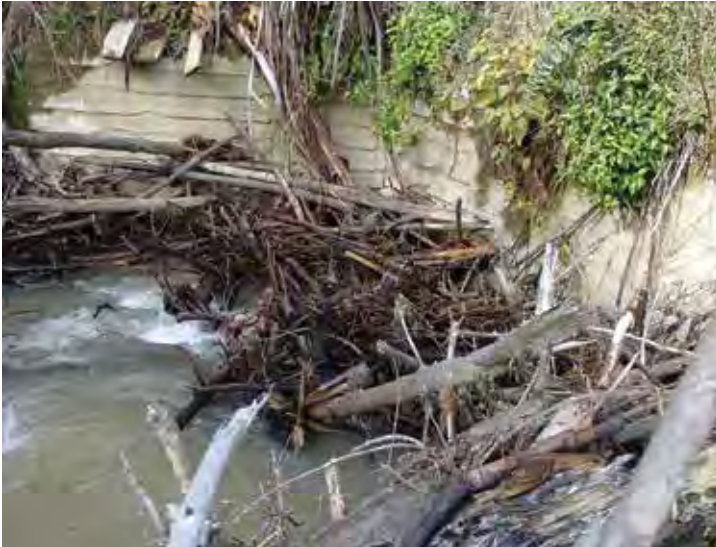
Left: Routine woody debris removal from a culvert inlet. Right: This unacceptable construction job has led to a major repair and maintenance problem. Uncompacted fill and poor inlet armouring will lead to unnecessary maintenance, NES-PF non-compliance and environmental risks
