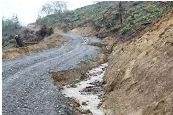
Left: A functioning ditch after heavy rain. Right: A heavily scoured ditch that has bypassed the culverts. Rock armouring and appropriate culvert spacing would have limited the impact
