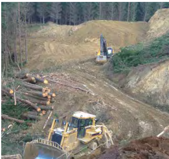
A 37t bulldozer (D8) and a 30t excavator constructing a new road and landing
