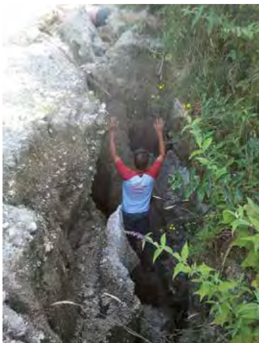
Check ditches for scour. Poor water control maintenance, along with heavy rain and a steep road section, created this bad mix of environmental, health and safety, and infrastructure risk in pumice country
