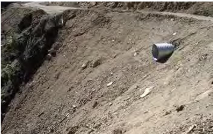
Flumes are needed to reduce fill scour or fill failure. This unprotected outlet will become an issue on the first rain then become an on-going problem
