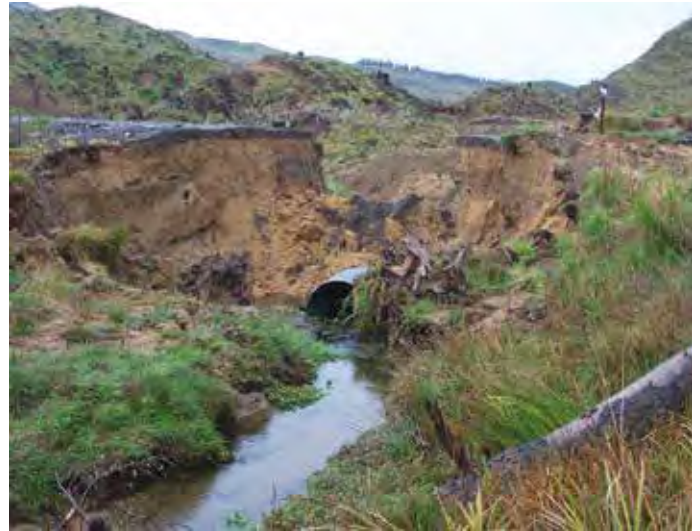
Left: A well-functioning spillway that protected the road when logging debris, mobilised by a 1-in-50-year storm, blocked the culvert mouth. Right: An expensive, inconvenient problem with potential environmental and downstream impacts. This pipe culvert failed when it was blocked by woody debris
