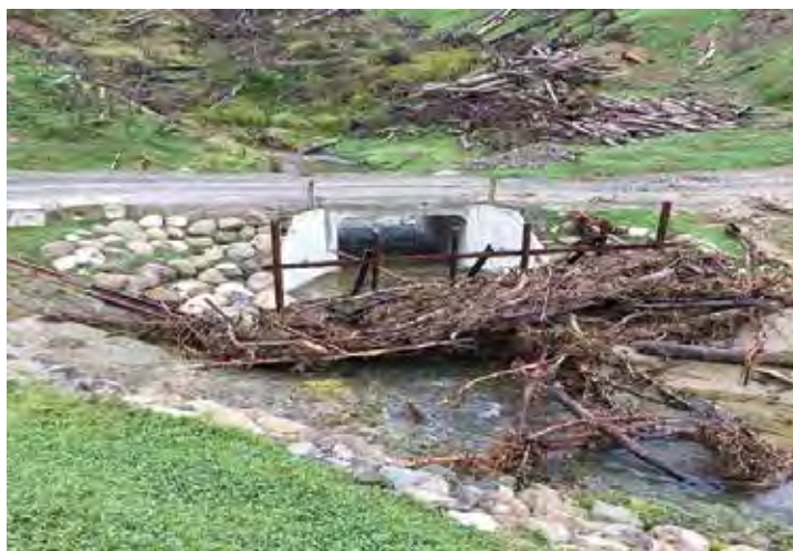
Left: An effective slash trap. Right: Effective slash trap installed upstream of road and bridge. An accessible site allows removal of slash and maintenance of the debris trap
