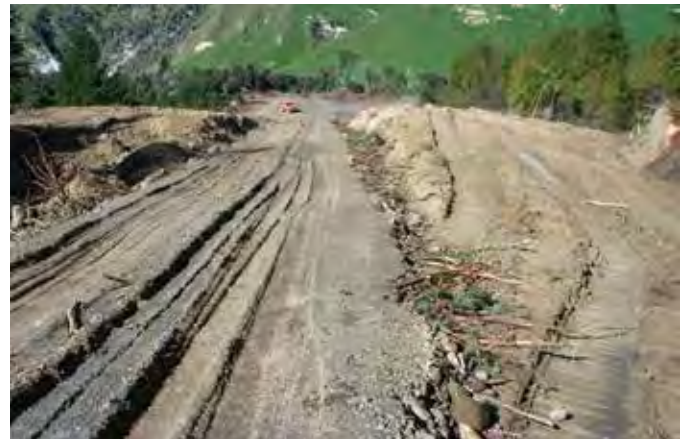
Slash corduroy provided truck access on a steep section of road after the subgrade failed
