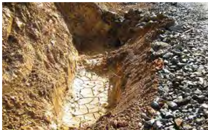
Left: A good example of a sediment trap with minimal ground disturbance and provision of an outlet. Right: There are sediment traps at both the inlet and outlet of this culvert. Immediately below the outlet is a waterway
