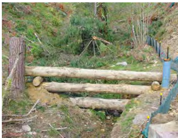
Left: These small traps were constructed to limit debris crossing from the forest into the adjoining property. Right: Logs can be an easy and effective option in this situation
