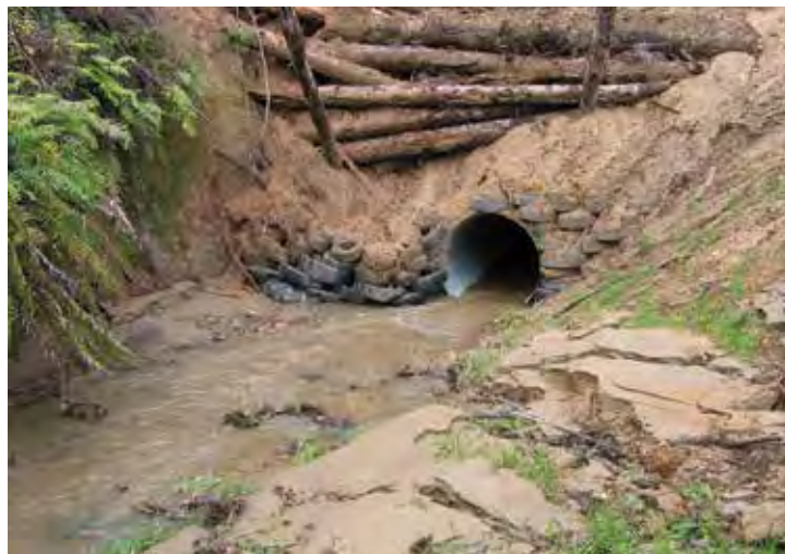
Left: This culvert needed a retro-treated log retaining wall to prop up the vertical fill slopes. Right: Again, the culvert was too short. And the 'fix' has failed. Tyres and untreated radiata logs are not acceptable for culvert armouring, because radiata rots rapidly, and tyres can readily move downstream if the structure loses integrity
