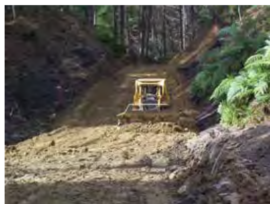
Above: Balancing cuts and fills help minimise the overall earthworks required to construct a forest road
