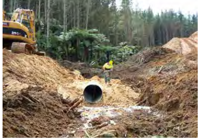
Left: Construction showing a temporarily diverted river. Right: Culvert installed on hard material with the fill being compacted. Note that the culvert appears to be perched in the photo, but it is not. Always consider the fish passage
