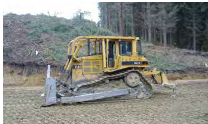
Track rolling will produce an attractive surface finish but has negligible compaction effect
