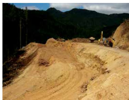
Below: Landings can generate large volumes of earthworks. Benching is essential in anything other than the easiest country to help stabilise the fill
