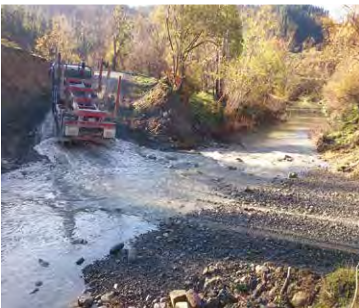
Left: Log truck using a natural ford crossing. Note that sediment comes from mud on the tyres, river bed disturbance, and displaced water that washes over the approaches and back into the river. Right: A concrete pad ford reduces sediment but can be a barrier to fish passage
