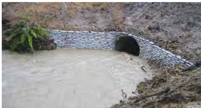
The large culvert with bagged cement and sandbag headwall has been designed to resist scour in debris laden flood flows
