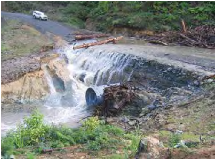
Left: A well-functioning spillway that protected the road when logging debris, mobilised by a 1-in-50-year storm, blocked the culvert mouth. Right: An expensive, inconvenient problem with potential environmental and downstream impacts. This pipe culvert failed when it was blocked by woody debris
