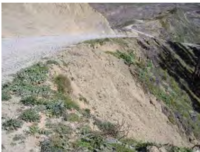
Left: Lack of a berm to control stormwater discharge over vulnerable fill has caused fill failure and sediment loss. Right: Overlarge berms create additional risk. An enlarged berm has been constructed to store excess material from cut banks. This has spilled down the fill slope to the water way in the gully. Despite compacting, the fill is now unstable and showing signs of collapse
