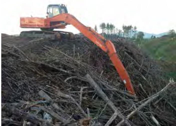
Top, centre, above: A landing failure reduces site productivity, and can trigger environmental effects like highly erosive debris flows. Large boom excavators increase the reach and slash that can be removed. The landing (centre) has had a normal excavator complete the rehab but significant slash remains
