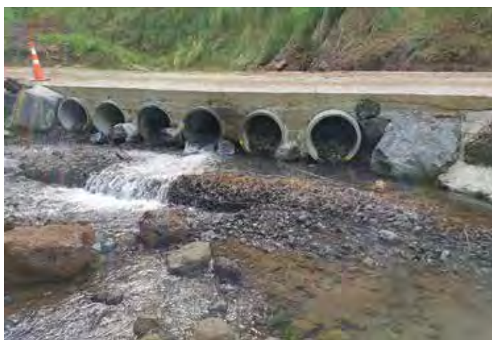
Left: The deflectors have effectively limited the amount of woody debris caught in the structure. Right: The reno mattress has protected the same crossing from being undermined, but could cause a fish passage issue if not addressed
