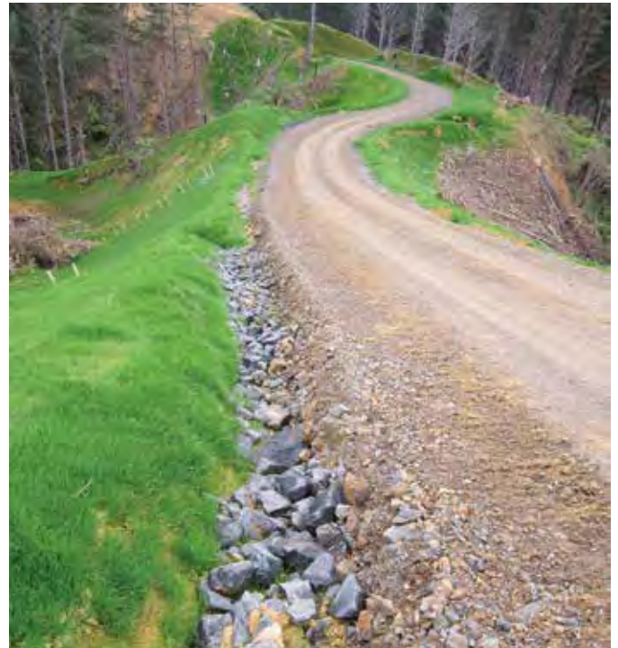
Above: An uncompacted berm vulnerable to sediment loss and failure. Right: A well-constructed berm with rock armoured ditch, hydroseeding and a slash bund at the base of the fill to contain sediment. A flumed cut out has been used to convey runoff over the fill. This berm will help protect the road and limit sedimentation
