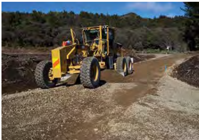
Grader reshaping road pavement
