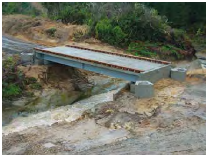
Left: Bridges can become part of a debris flow even in a well-sited location. Make sure the bridge soffit is at least 1 m above a 2% AEP event. Right: The replacement is a metre higher
