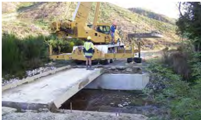
A crane will be needed to install and remove the structures
