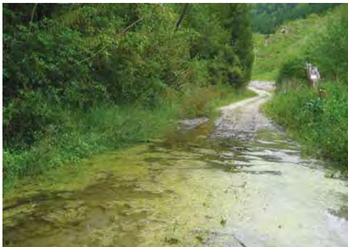
Insufficient ditch depth plus poor shoulder maintenance led to water following the road
