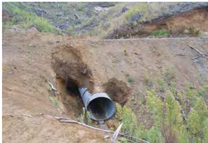
Left: Ensure provision of adequate cover of compacted fill over the pipe. Right: Poor compaction during culvert installation has led to failure as water is now bypassing the structure
