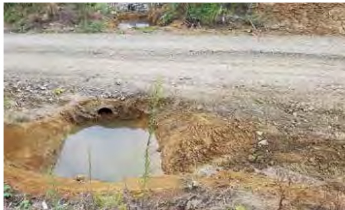
Left: Making sufficiently effective sediment traps is challenging in steeper terrain. This one is a potential safety concern as it is encroaching on the roadway. Right: Although this trap has worked, it is too small and not deep enough below the culvert mouth
