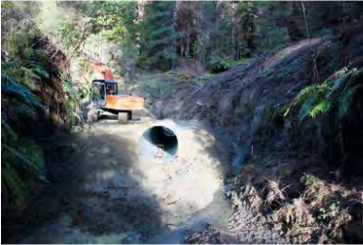
Left: Construction showing a temporarily diverted river. Right: Culvert installed on hard material with the fill being compacted. Note that the culvert appears to be perched in the photo, but it is not. Always consider the fish passage
