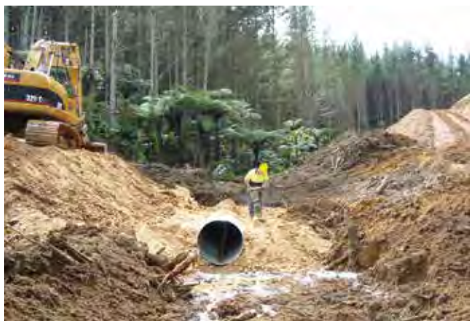
Compacting fill material around a culvert is important to avoid failure in the long term
