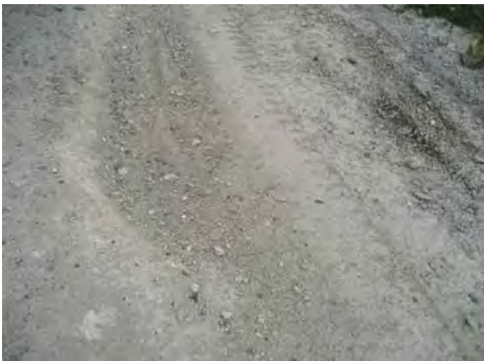
Pavement showing a soft spot
