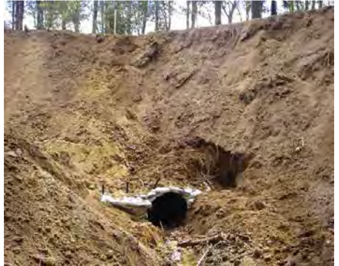
Left: Routine woody debris removal from a culvert inlet. Right: This unacceptable construction job has led to a major repair and maintenance problem. Uncompacted fill and poor inlet armouring will lead to unnecessary maintenance, NES-PF non-compliance and environmental risks
