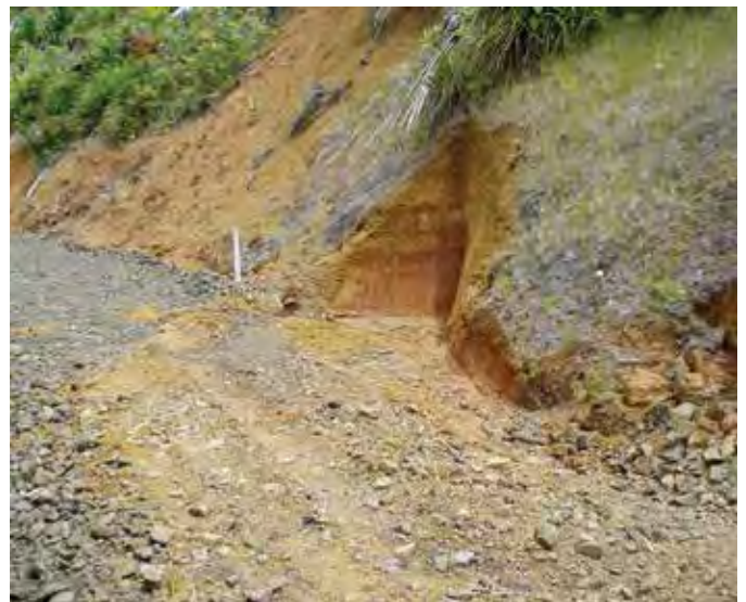
A typical drainage culvert inlet with a sediment trap before it. The trap is deeper than the pipe inlet, and it can easily be cleaned out by an excavator
