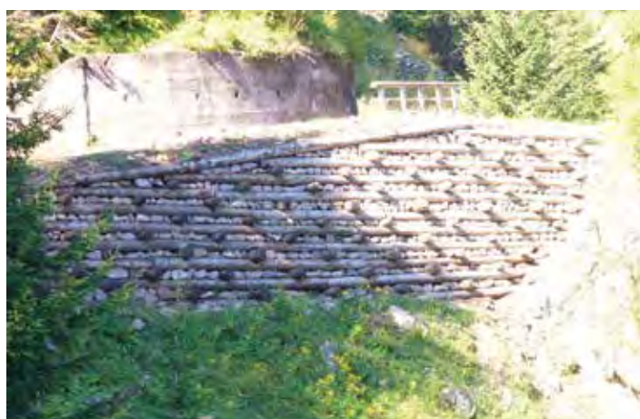
Treated timber crib as retaining wall of forest road fill slope. Never use untreated radiata logs as they are not durable
