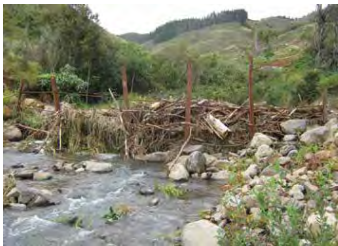
Left: An effective slash trap. Right: Effective slash trap installed upstream of road and bridge. An accessible site allows removal of slash and maintenance of the debris trap
