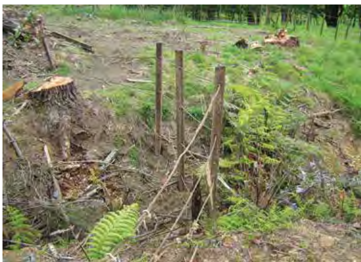
Left: These small traps were constructed to limit debris crossing from the forest into the adjoining property. Right: Logs can be an easy and effective option in this situation
