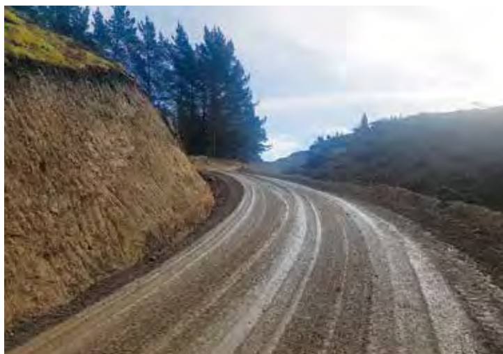
Left: Scouring can rapidly occur during heavy rain. Right: Good crossfall helps reduce scouring
