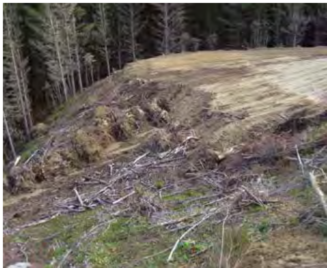
Stumps have been placed on a bench, which is a safe location and one that will not cause environmental issues
