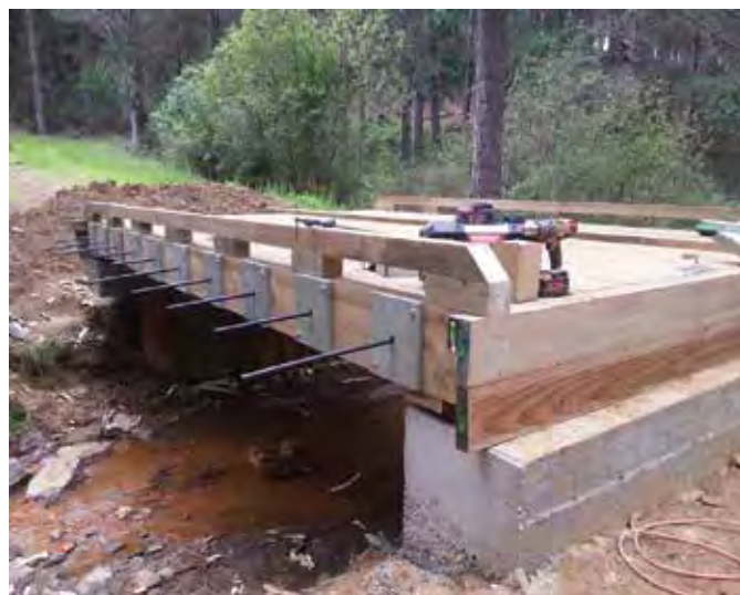
An option to concrete and steel – a New Zealand designed composite post-tensioned treated wood composite bridge
