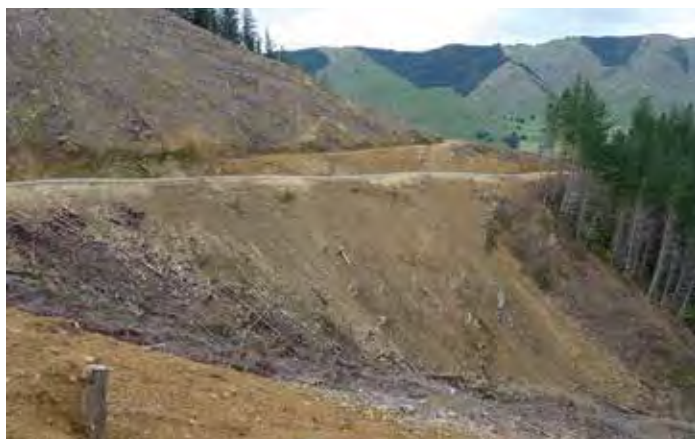
Left: While side casting is often the easiest way to build a road, the material pushed over the edge onto the slope is very susceptible to erosion and failure. Right: Tension cracks have developed on the landing. Over time it will allow water to infiltrate and cause the fill slope to slump. It is very important to correctly bench and compact fill material
