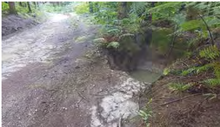
Left: Making sufficiently effective sediment traps is challenging in steeper terrain. This one is a potential safety concern as it is encroaching on the roadway. Right: Although this trap has worked, it is too small and not deep enough below the culvert mouth
