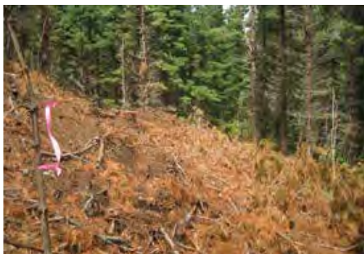
Re-establishing the grade line after road line salvage using taped branches as markers
