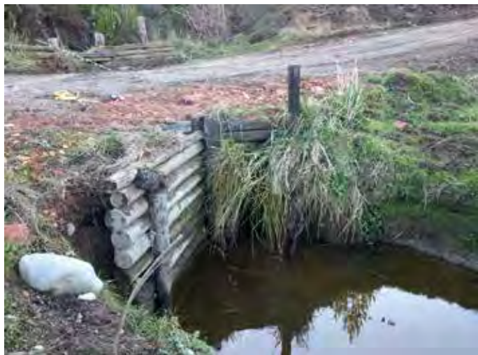
Left: This culvert needed a retro-treated log retaining wall to prop up the vertical fill slopes. Right: Again, the culvert was too short. And the 'fix' has failed. Tyres and untreated radiata logs are not acceptable for culvert armouring, because radiata rots rapidly, and tyres can readily move downstream if the structure loses integrity
