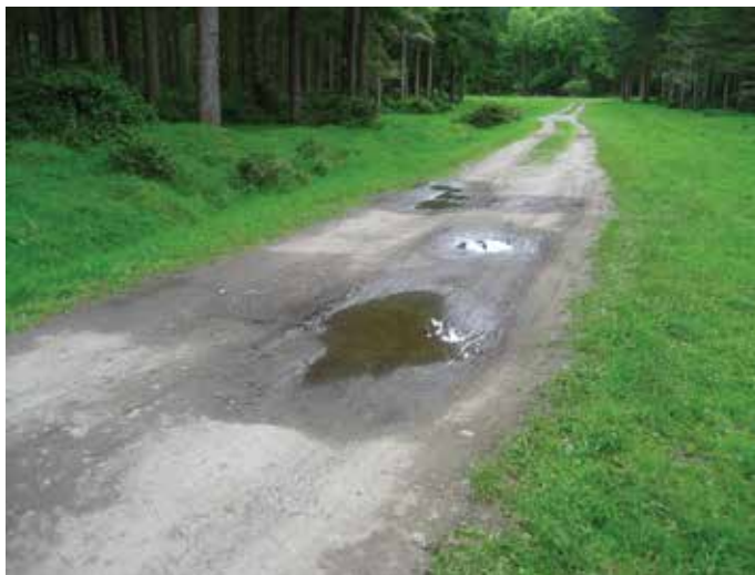
Potholes retain water that penetrates the aggregate, causing a further reduction in strength
