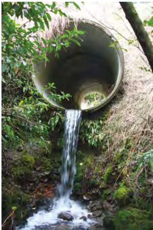
A perched projected culvert eliminates fish passage
