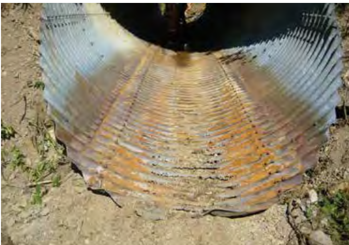
A rusted-through steel culvert floor and a concrete pipe's floor worn past its steel reinforcing
