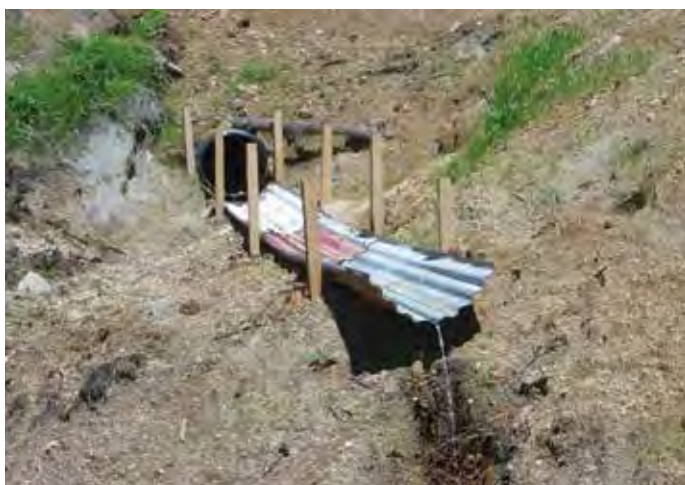
Left: Galvanised iron or tin flumes are not good practice. They increase water speed, and cannot easily follow the terrain. The sheets do not lock together, and can fall apart. Right: Rock armouring cut-outs and culvert exits are an effective way to reduce water speed and scouring
