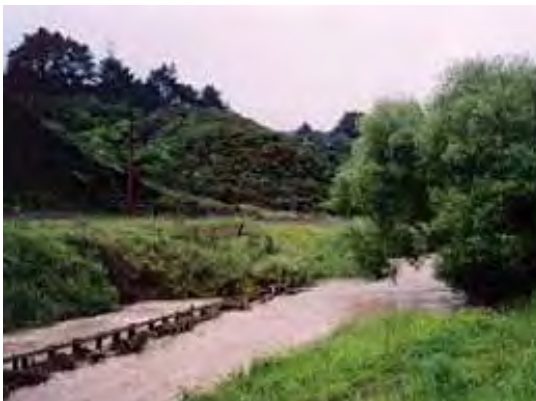
Left: A tapered debris retention fence during heavy rain. Note the debris trapped in the structure. Right: Post clean-up
