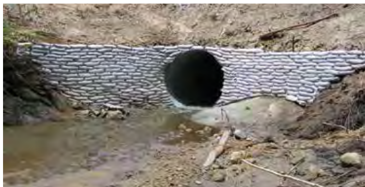
The large culvert with bagged cement and sandbag headwall has been designed to resist scour in debris laden flood flows
