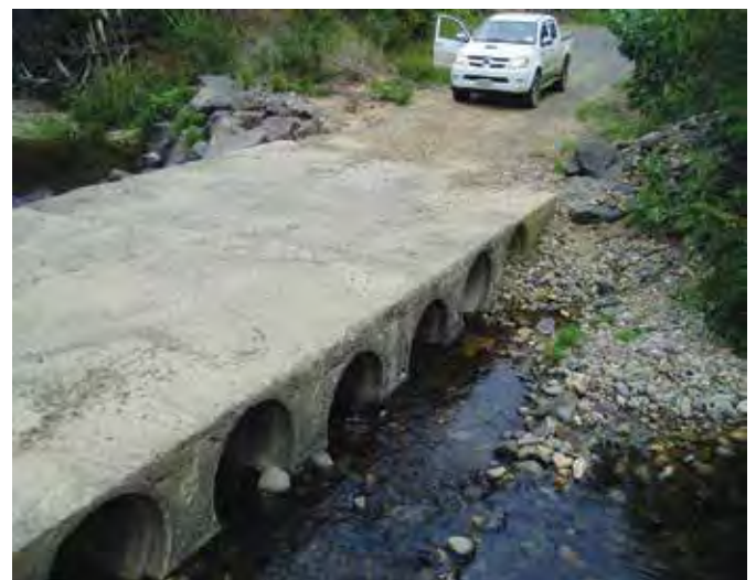
This battery culvert provides for fish passage
