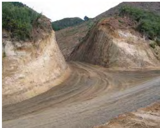
Papa/mudstone can have steep batter slopes which also reduce the volume of material that needs to be moved
