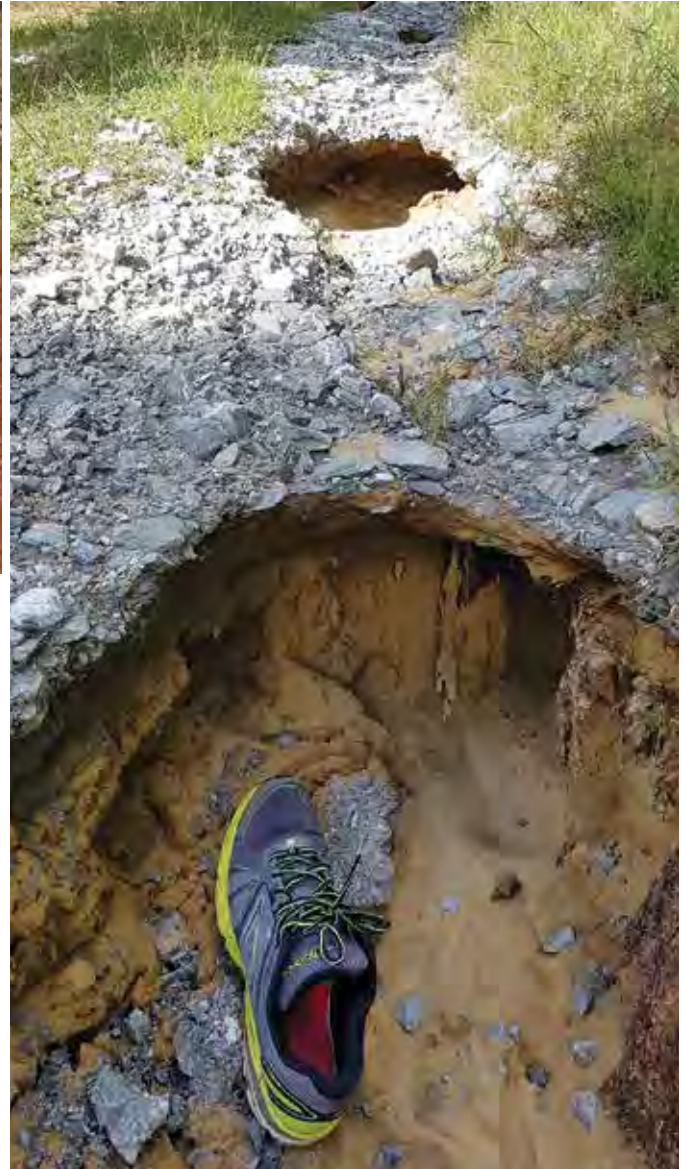
Left: Rock armour using subgrade aggregate. Right: Rock armouring is effective, however, in this instance, the rock was not deep enough in parts to stop scouring
