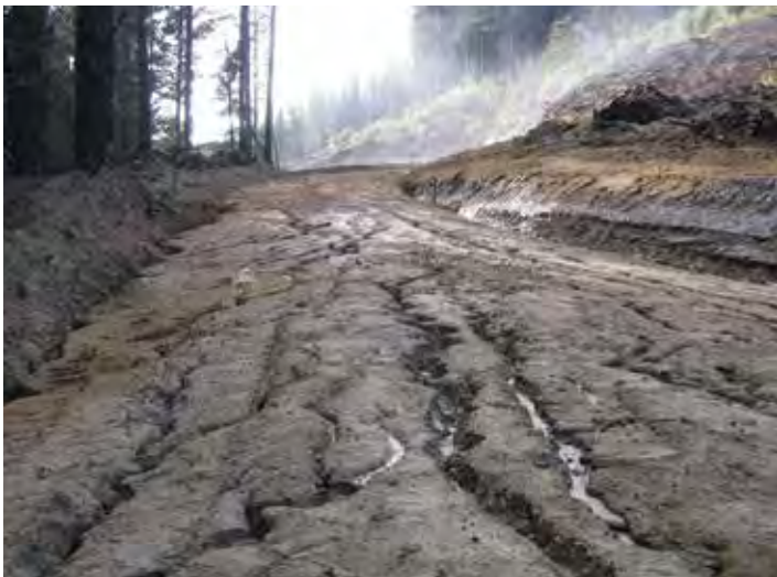
Poor water control during construction can damage a road and cause severe erosion
