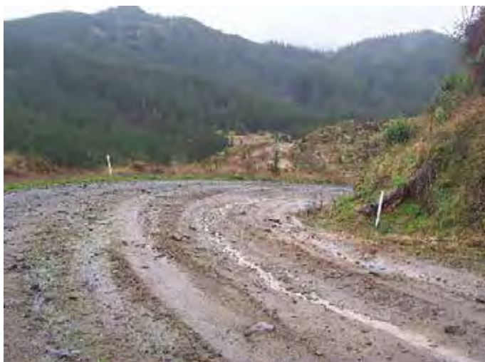
Left: Scouring can rapidly occur during heavy rain. Right: Good crossfall helps reduce scouring
