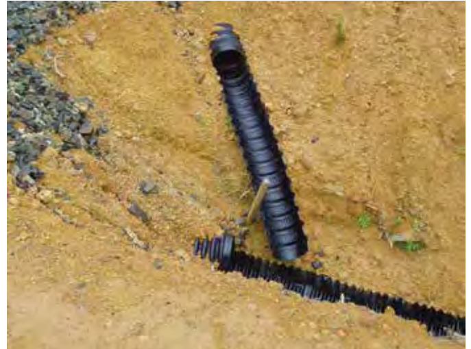
Above: Many components in this image are poor practice. The flume entrance is likely to be bypassed, the flume is poorly pegged, and debris from the slope above is already rolling into the lower flume and partially blocking it. This will create infrastructure and environmental risk.
