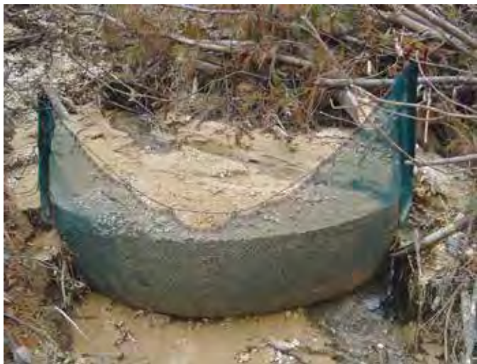
This fence needs maintenance. Sediment is spilling around the sides of the structure
